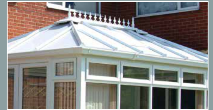
TRADITIONAL CONSERVATORY ROOF
